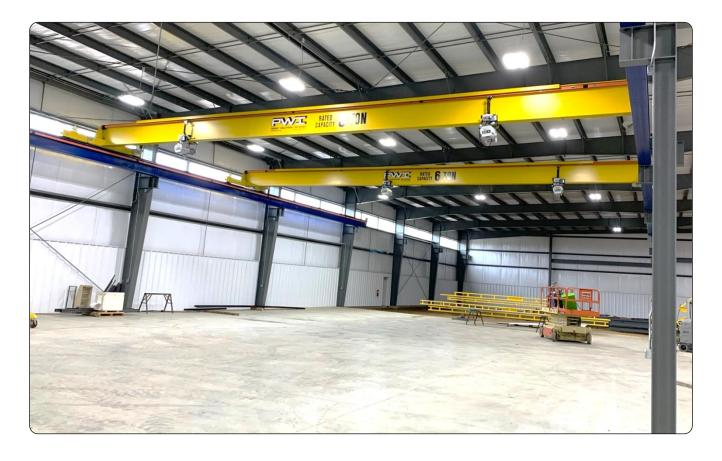
Motorized Top Running Single Girder Bridge Crane
