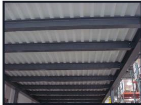
B-Deck- The wider spaces between ribs of the decking is toward the top.
